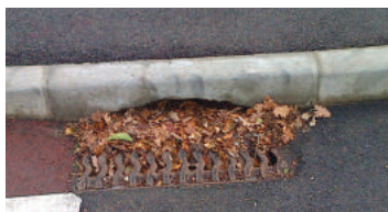
Avaloir - Source : ATTF
